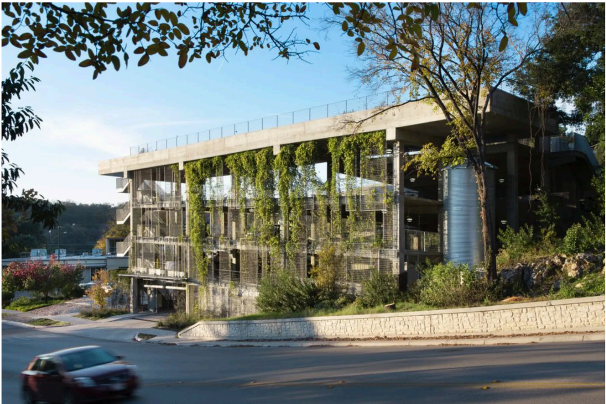
T3 Parking Structure | Danze Blood Architects
